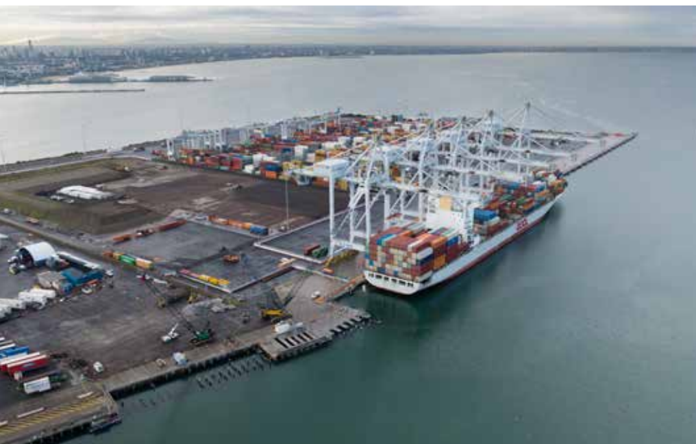
Webb Dock East Extension Project
